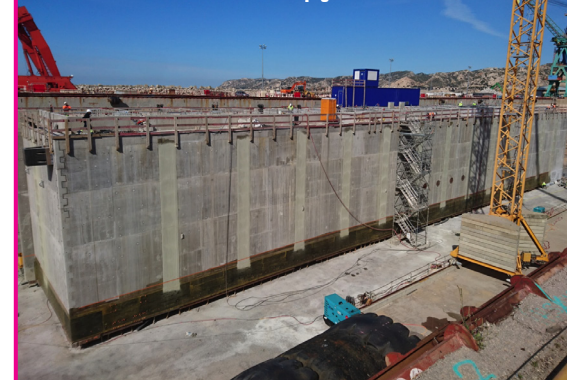
Seal fitted at the base of the ship gate
